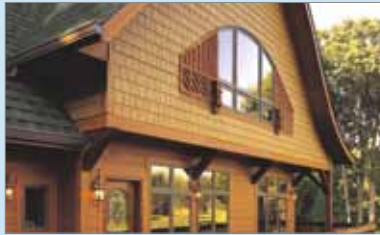
Fiber Cement Siding
