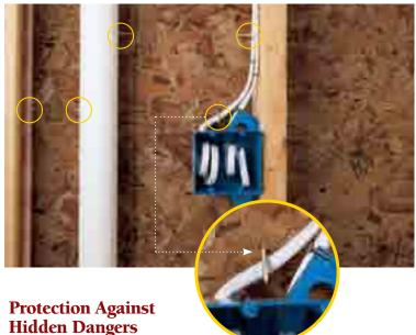
Precise installation contributes to wind load performance, and helps avoid nailing into anything located between the studs, like plumbing or wiring that could create a number of dangers...
